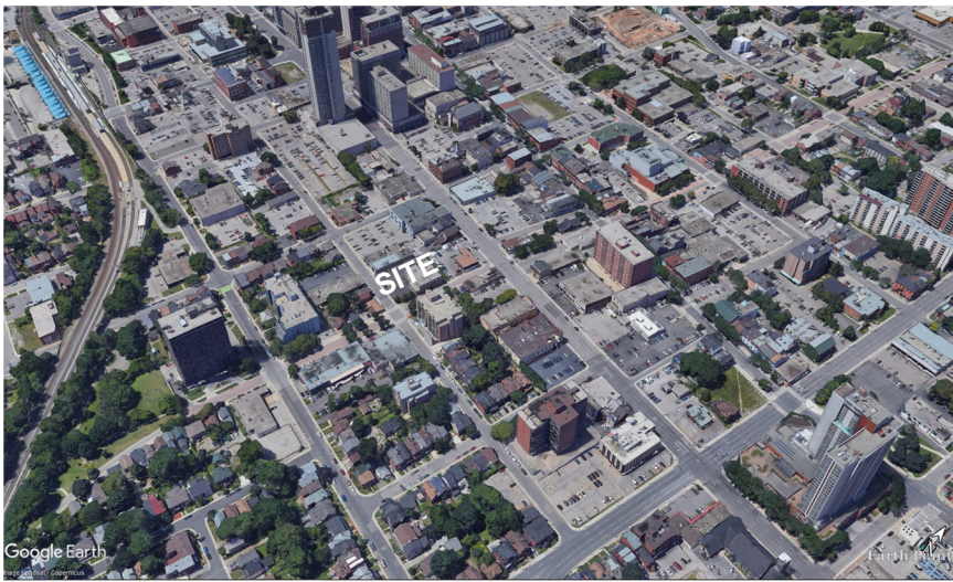
View of the area subject to morning and mid-day shadows – Looking West
