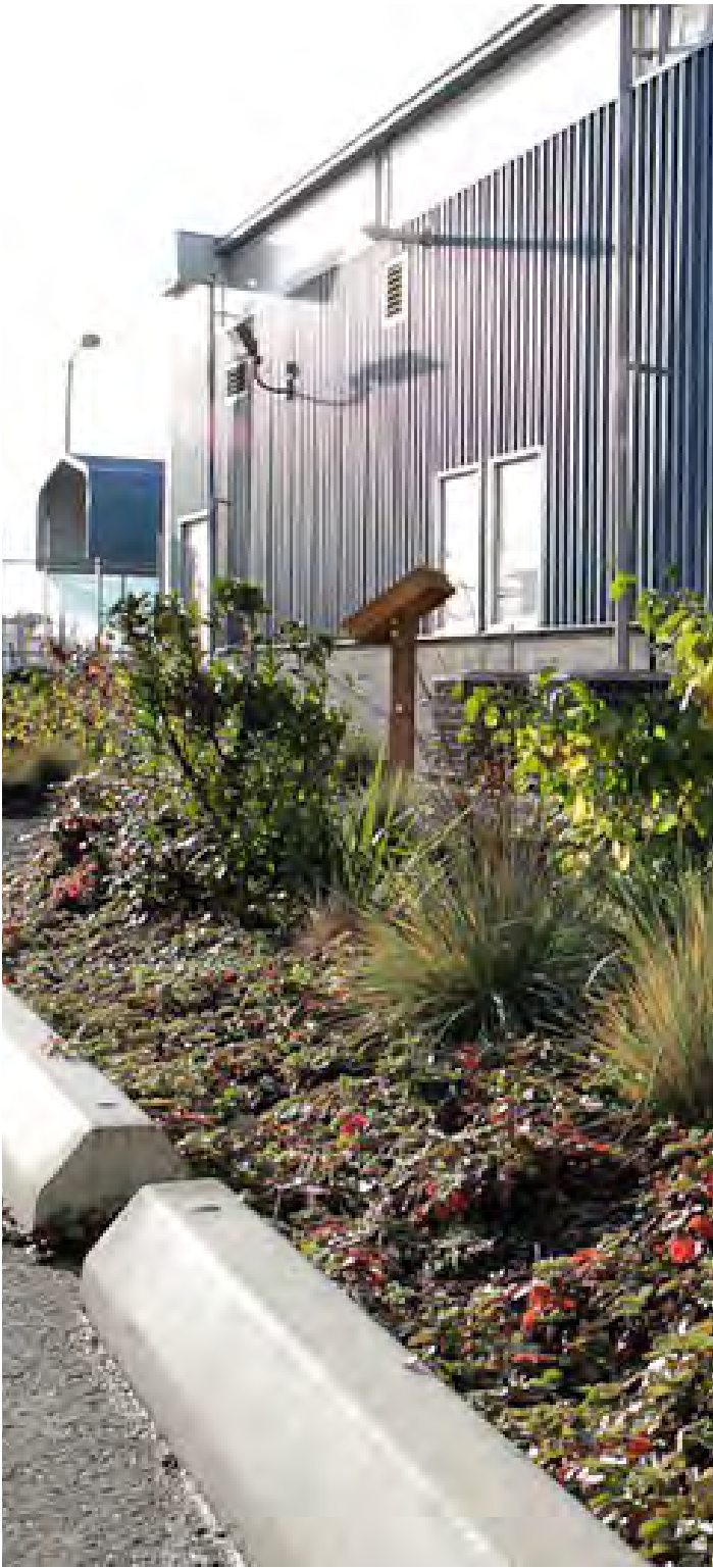
Example of an industrial rain garden, Totem Ocean Trailer Express, Tacoma, WA. Credit: Katie Campbell
