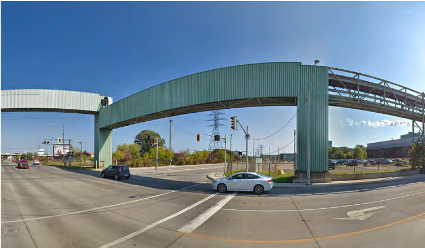
Existing Condition at Kenilworth Ave N. and Dofasco. Credit: City of Hamilton
