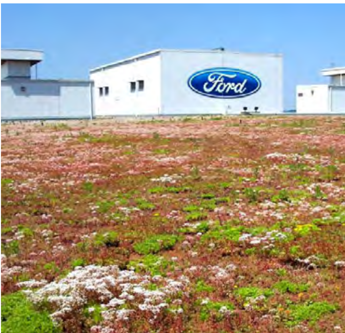
Example of reduction of hardscape to improve site filtration, Ford Motor Company Factory Green Roof, River Rouge, MI Credit: Xero Flor America, LLC
