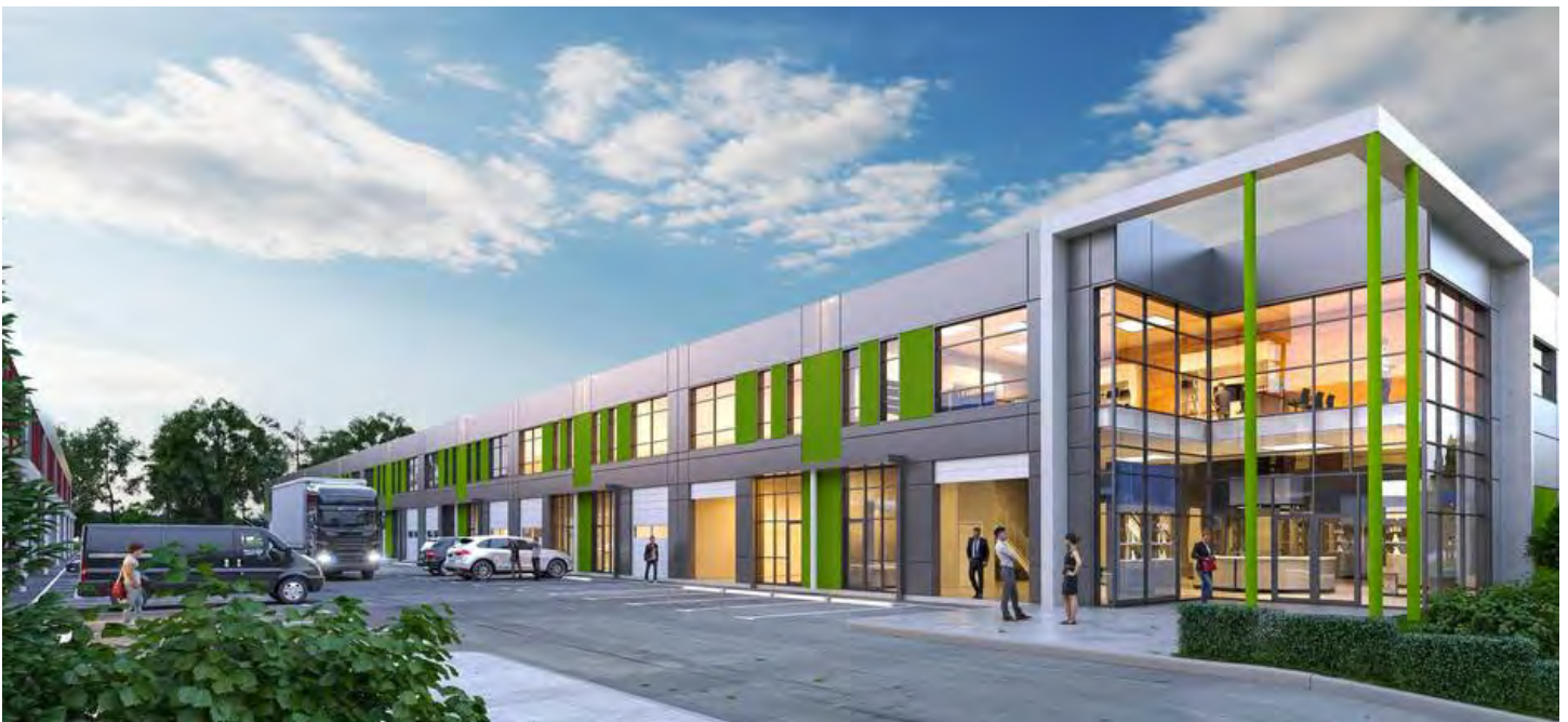
Example of high quality materials and architectural detail, IntraUrban Business Park. Vancouver, British Columbia Credit: PC Urban
