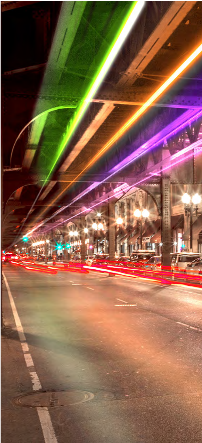
Example of revitalized space underneath overhead infrastructure, Wabash Lights. Chicago, Illinois. Credit: Jack C. Newell
