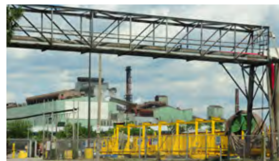
View of overhead industrial infrastructure. Credit: Dillon Consulting
