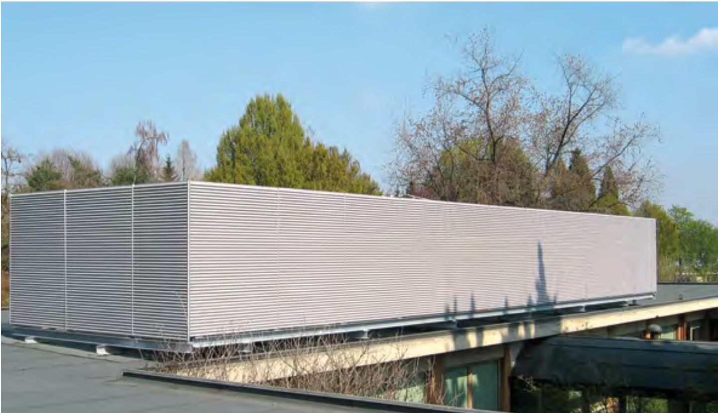
Louvered screening with galvanized steel. Credit: Lang and Fulton
