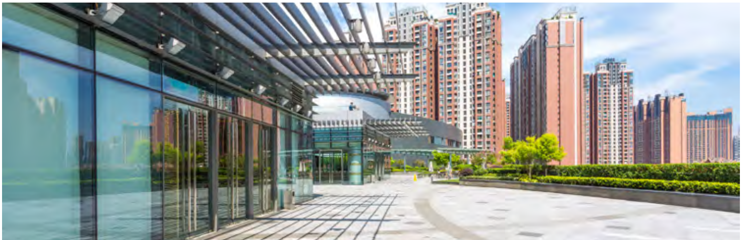
Building with shade structure. Credit: Zhu Difeng
