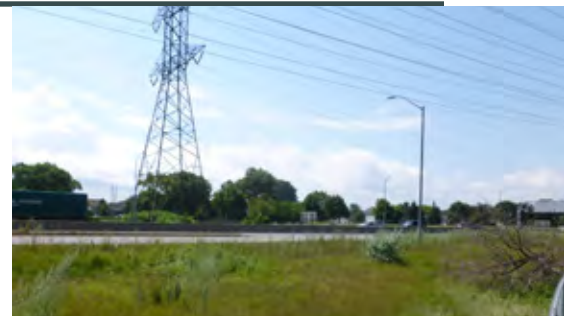
View of existing condition at east Gateway, Nikola Tesla Boulevard prior to the first instance of the split in expressway and collector road infrastructure. Credit: Dillon Consulting
