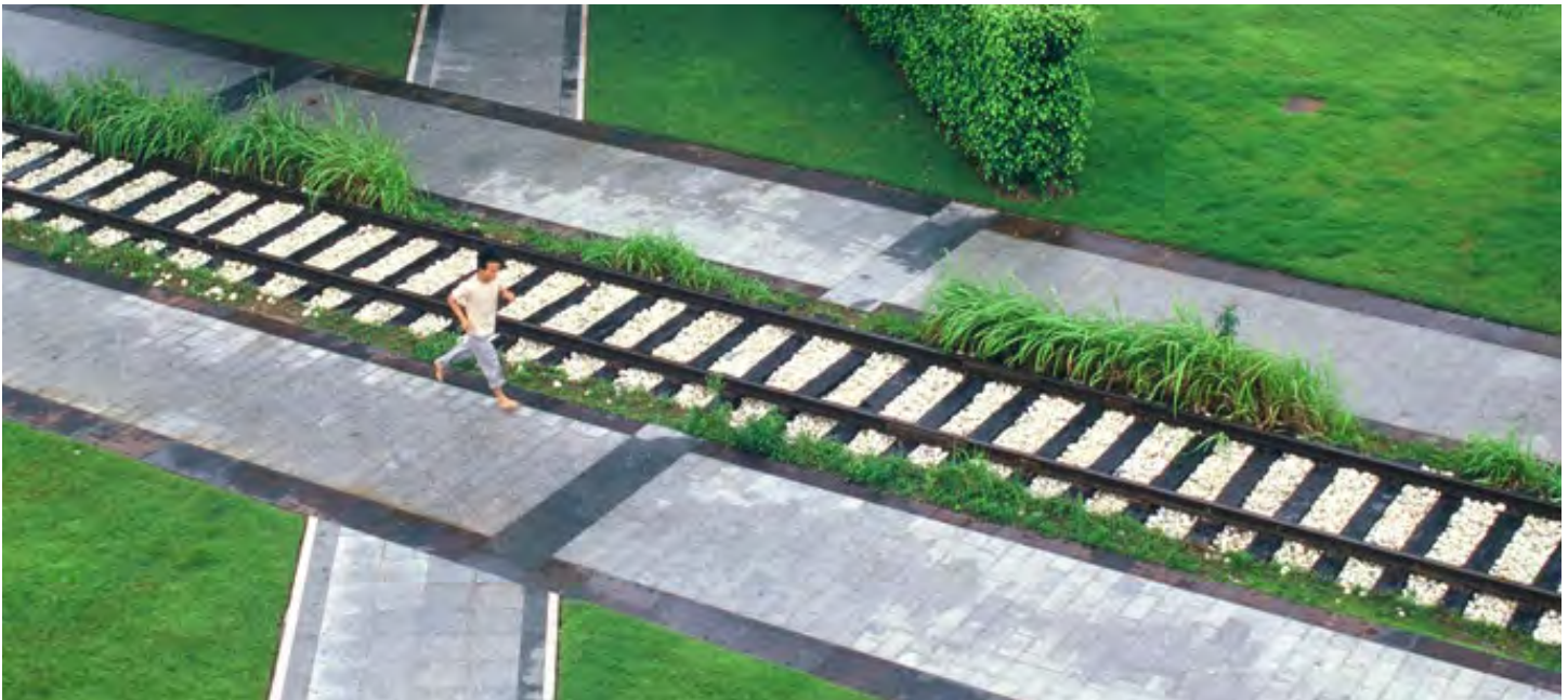
Respecting existing character, built form and landscape where appropriate, Zhongshan Shipyard Park. Zhongshan City, Guangdong Province. Credit: Kongjian Yu, Yang Cao
