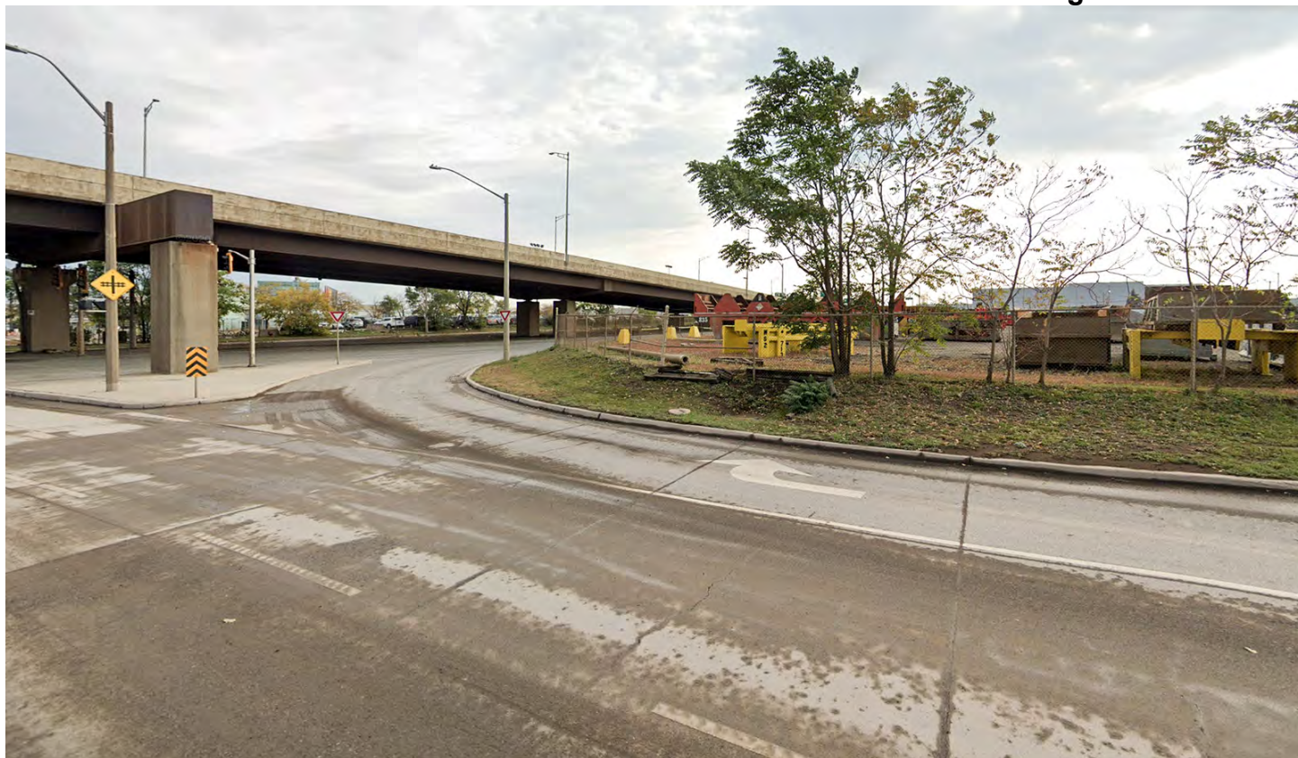
Existing Condition at Kenilworth Ave. N and Burlington St. E. Credit: City of Hamilton
