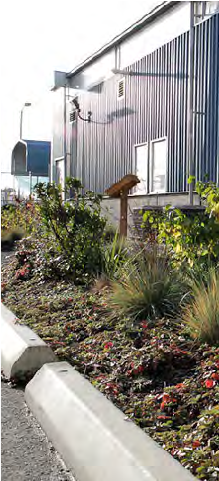
Example of an industrial rain garden, Totem Ocean Trailer Express, Tacoma, WA. Credit: Katie Campbell
