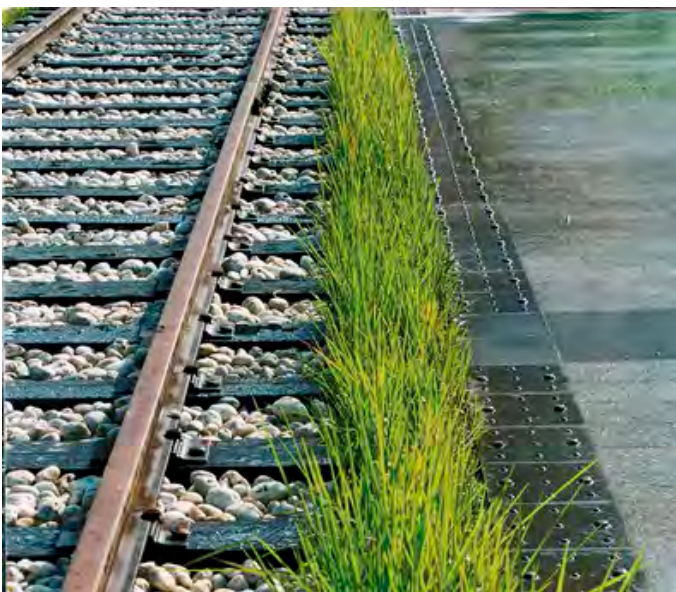
Example of clear separation between motorized and non-motorized movement, Zhongshan Shipyard Park. Zhongshan City, Guangdong Province. Credit: Turenscape
