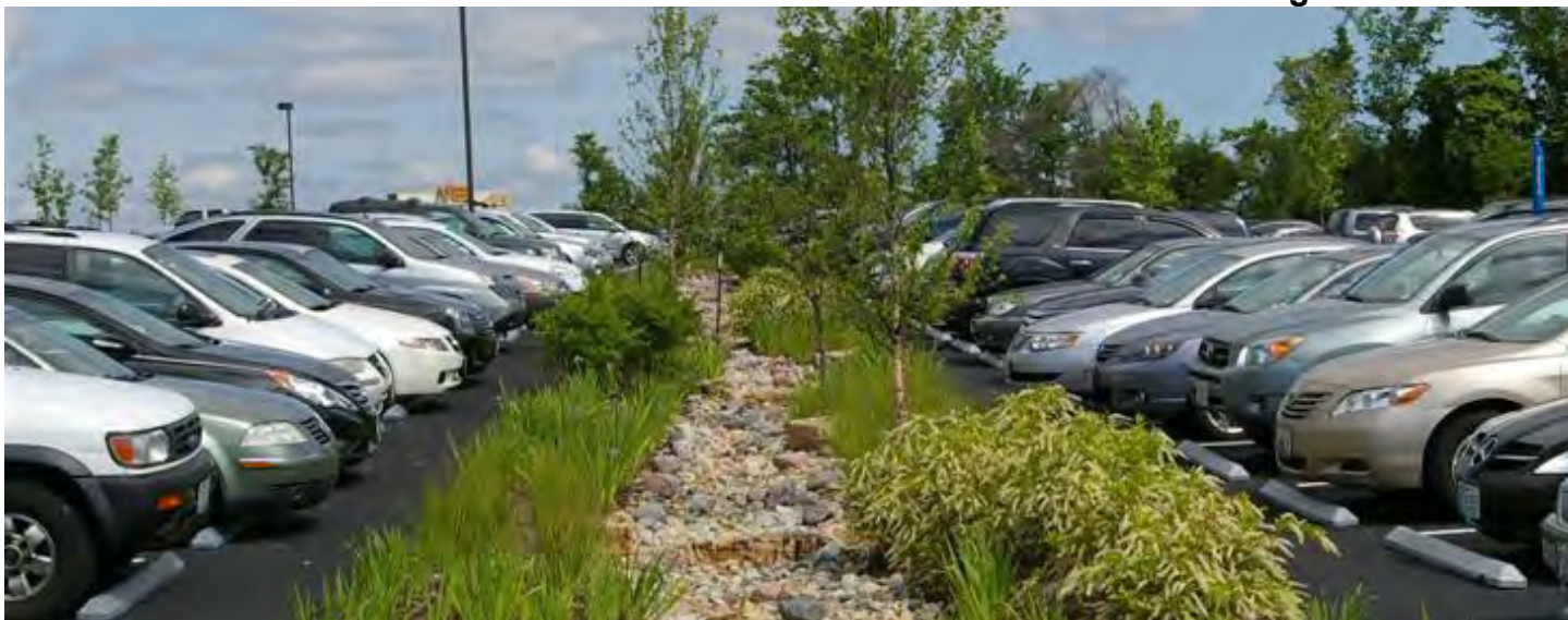
Parking lot with swale, Kimberling Shopping Center, Kimberling City, Missouri. Credit: Grownative.org
