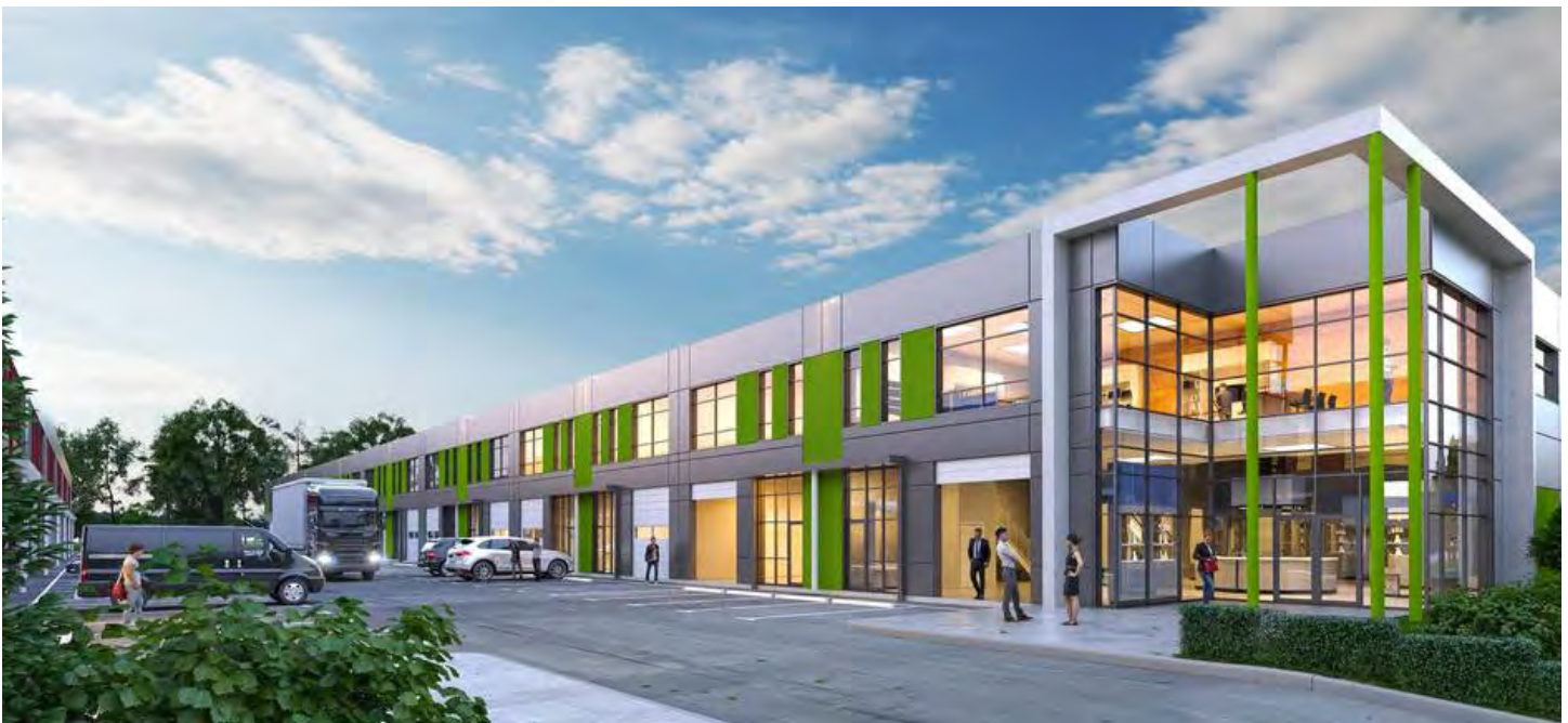
Example of high quality materials and architectural detail, IntraUrban Business Park. Vancouver, British Columbia Credit: PC Urban
