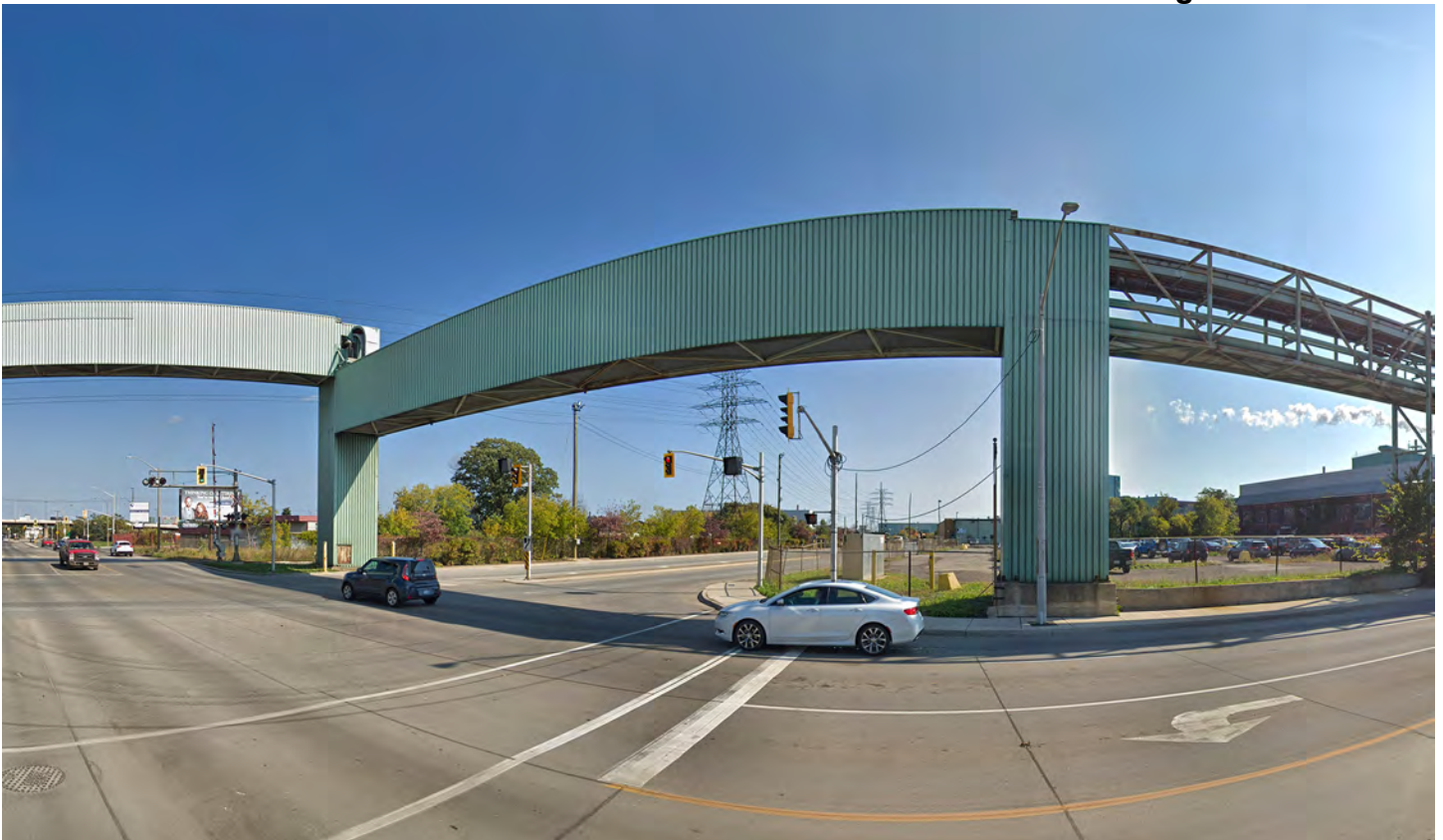
Existing Condition at Kenilworth Ave N. and Dofasco. Credit: City of Hamilton
