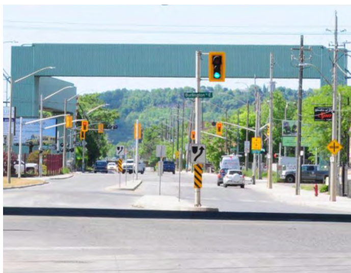
View of the escarpment and industrial infrastructure from Burlington Street East. Hamilton, Ontario. Credit: Dillon Consulting
