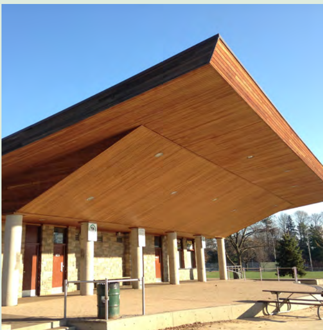
Figure 29: Washroom facility at the Dundas Driving Park
