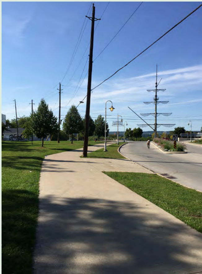
Figure 11: Multi-use boulevard trail along the south side of Strachan St. W. between Bay St. N. and James St. N.
