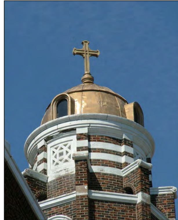
St. Stanislaus Roman Catholic Church Copper Cupola
